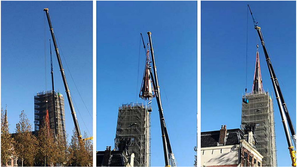
The new spire being placed on the Saint Laurentius Church, 8 November 2016. Photos by NH.
