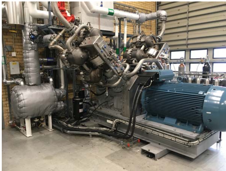
Fig. 1. The HighLift Stirling-cycle-based heat pump (SC HP) from Olvondo Technology is installed in the heat pump room at pharmaceutical company AstraZeneca, Gothenburg, Sweden. The nominal heat output from the heat pump is between 450 and 500 kW [6].
